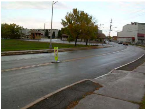
Figure 12 – Curb drop on Route 46&32 has no corresponding crosswalk or curb drop on other side of road.
