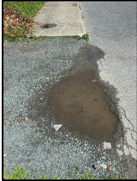
Figure 13. Ponding at the edge of a driveway along South Main St. South of Riverside Park South.
