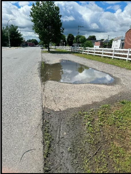
Figure 18. Ponded stormwater observed along the side of Railroad Street.
