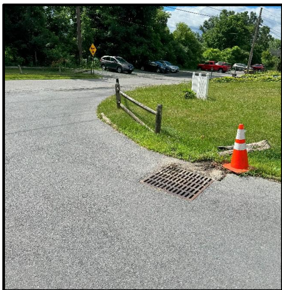
Figure 29. Close up of catch basin where stormwater ponds at intersection of Warsaw Ave and Mulberry Street.
