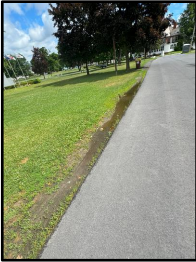
Figure 9. Flooding along the edge of Park Place and the grass at the park.
