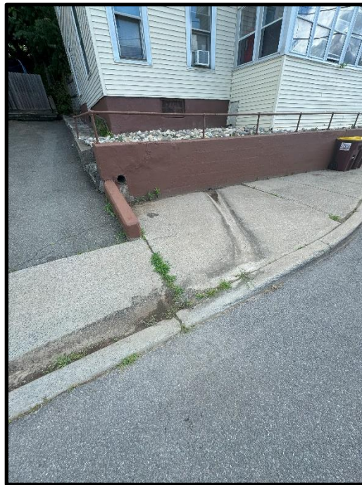
Figure 28. Area on the north side of the intersection of Warsaw Ave and Leonard Street where stormwater ponds.
