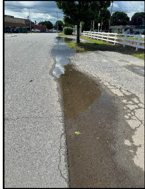
Figure 19. Ponded stormwater and “Alligator cracking” observed along the
