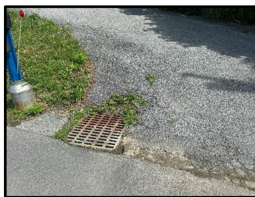
Figure 27. Close up of catch basin at end of residential driveway at intersection of Warsaw Ave and Maple Street.
