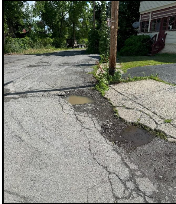
Figure 31. Pothole and “Alligator cracking” at North end of Penrose Ave.
