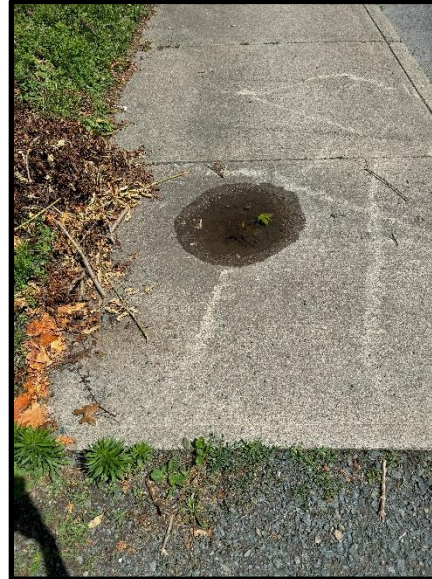
Figure 14. Ponding along the sidewalk along South Main St. South of Riverside Park South.
