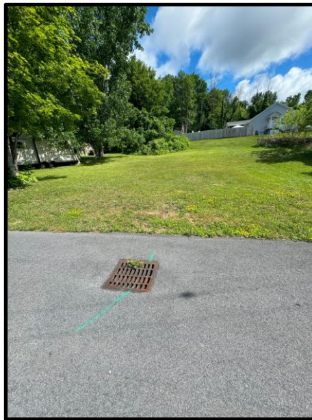
Figure 20. Catch basin on Walnut Street West of Pittsburgh Ave with the upgradient drainage area in the background.
